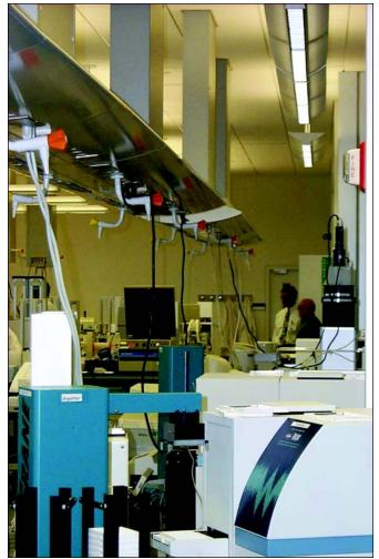
Figure 3. Overhead service carrier keeps services up and out of the way of mobile casework and carts underneath, yet handy for quick instrument connections.
