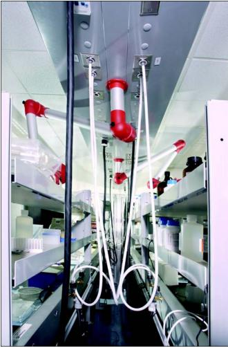
Figure 6. Quick-connect fittings are used on the overhead service carrier and the rear of the service manifold on the cart to simplify service connections when instruments are rolled into place.
